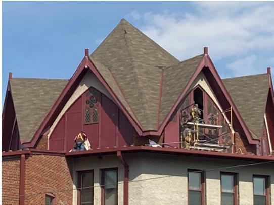
*Contractors work to remove Ballroom windows for restoration and temporarily board up the window openings.*
