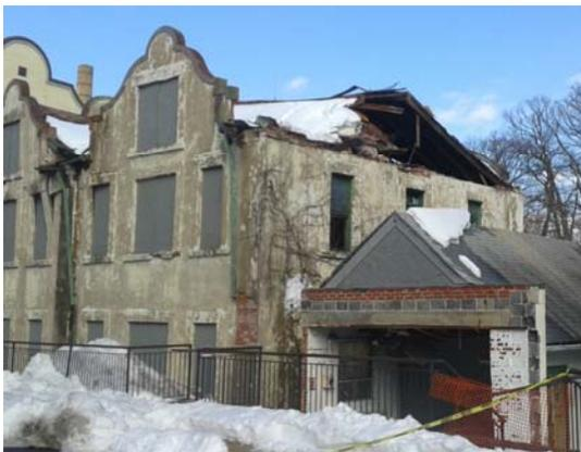
In the process of cleaning up the collapse, the owner/developer found that the remaining gables of the carpenter shop were not stable enough and thus had to be removed along with the complete roof to avoid further collapses. A temporary roof was built as soon as possible after the demolition and cleanup work was completed.
